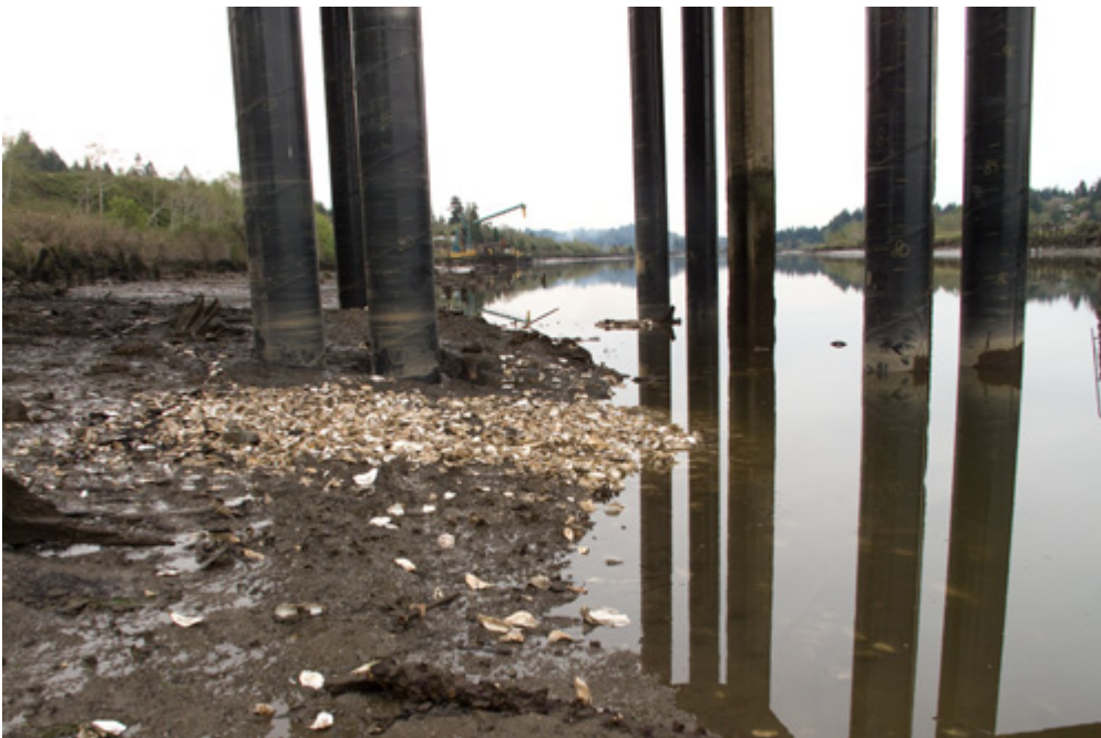
Figure 6: Post work view, most new shell below pictured tidal level
