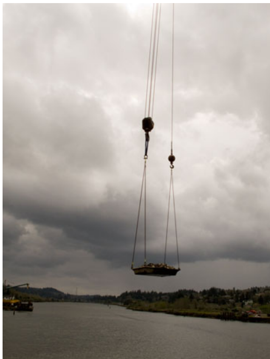
Figure 5: Crane moving shell material
