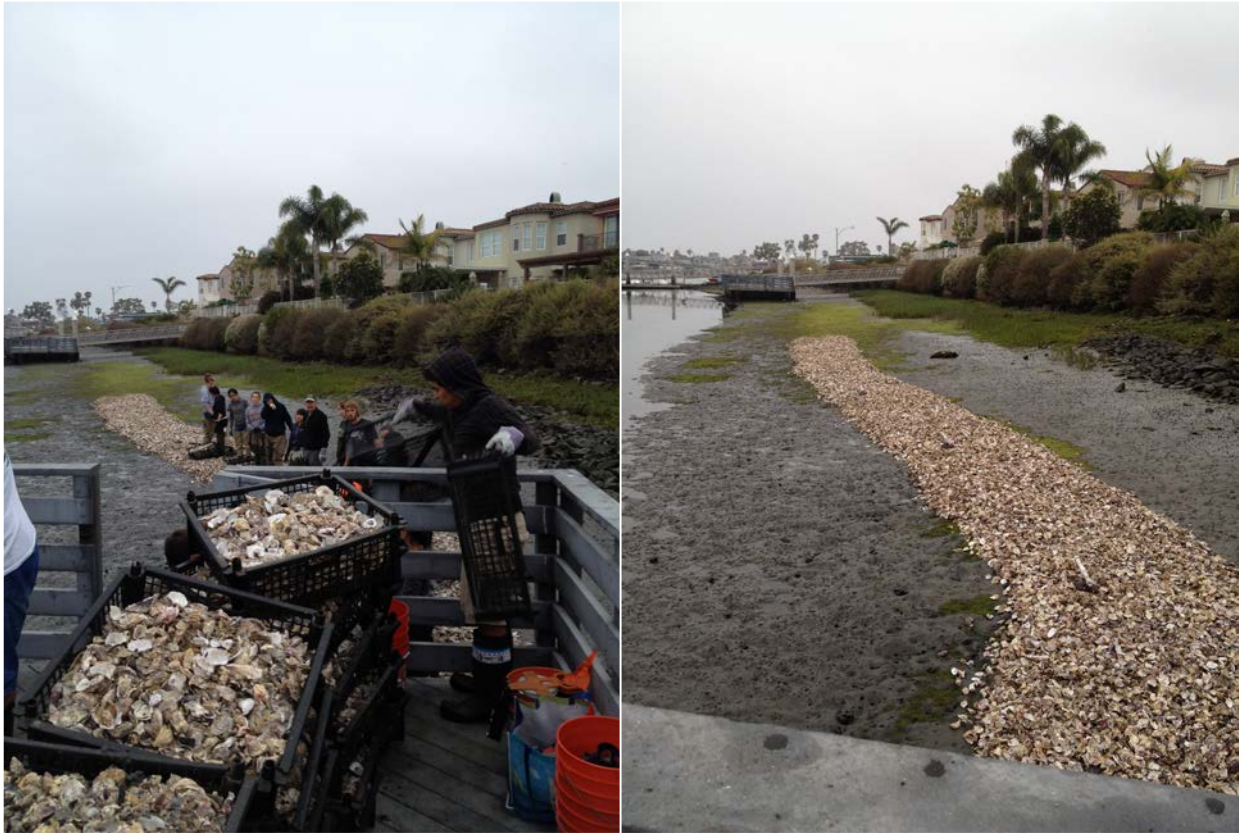
Figure 2. Left: Community volunteers construct the oyster bed in June 2012. Right: Completed bed, with control plot visible at same tidal elevation in the background.
