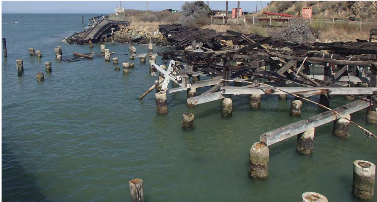
Failed northern section of the Richmond Terminal 4 pier revealing the principal construction of the pier to be short concrete wrapped wood piles supporting a lattice work of beams and cross members that held the pier deck. Deck support beams and encased piles both show evidence of creosote treatment.
