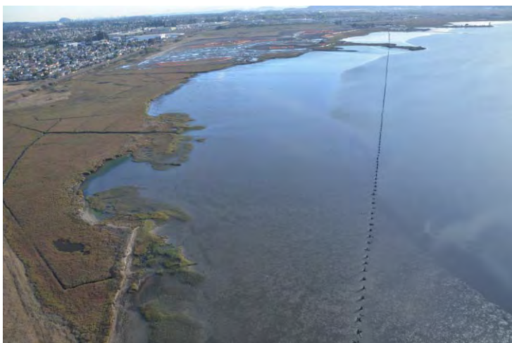
Low tide view of the pipeline trestle crossing intertidal mudflats
