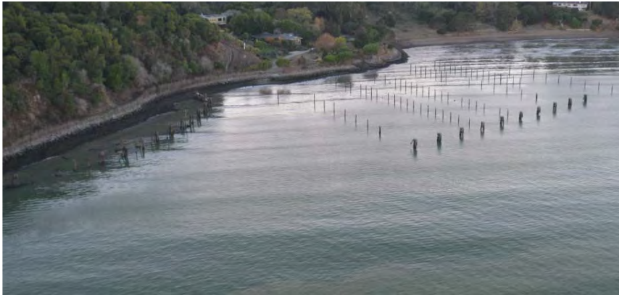
Aerial overview of the El Campo marina site illustrating the larger dolphin pile clusters along the shoreline and outboard of the marina pile field.
