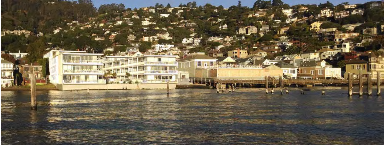
Current condition of the pile field at Sausalito 3 (Nunes Brothers Boat & Ways Company piers).
