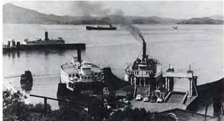
Photograph of the Castro Point terminal of the Richmond-San Rafael Ferry Company. The ferry docks in the foreground were located near the shoreline while the background pier is the present deteriorating ferry dock
