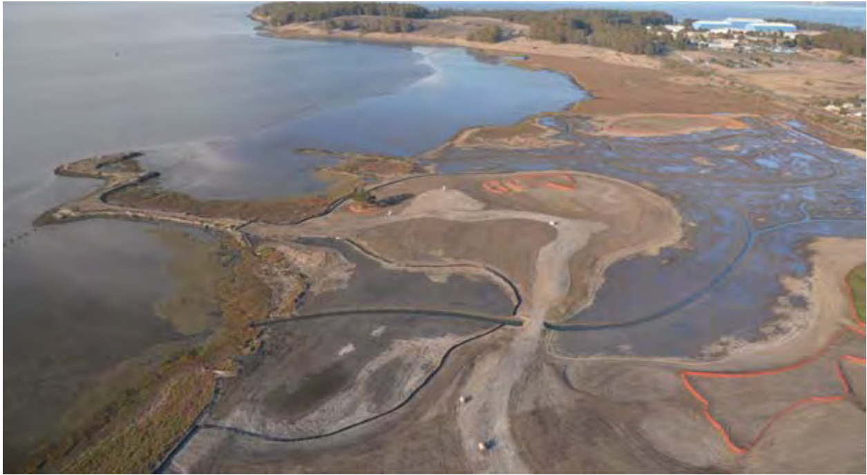
Upland access conditions to the pipeline trestle are not suitable through the Breuner Marsh (foreground) or Point Pinole Regional Shoreline (background).
